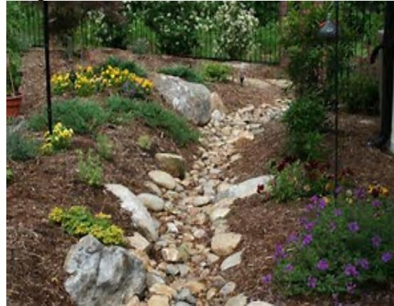
A SWALE slows down the rapid flow of stormwater runoff by ponding water between its sloping sides, often called berms.
